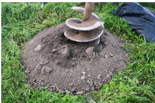
The augur was a Godsend – the 60 holes were dug with ease
